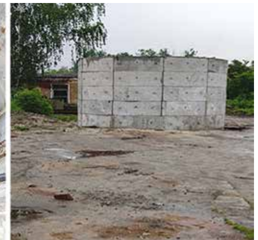
Figure 6.20. A pit shaft on Grekivska street
