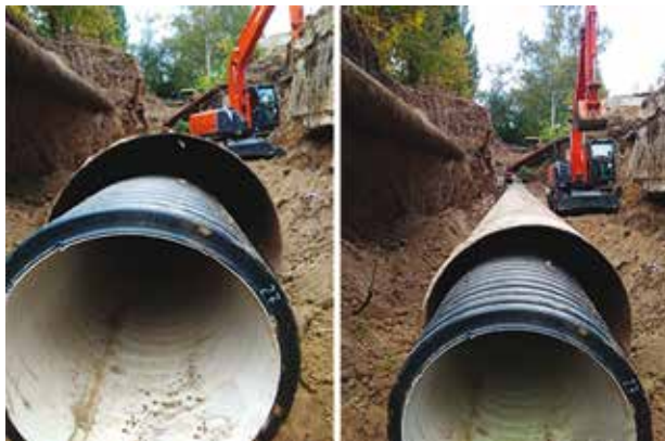
Figure 6.26. Rehabilitating \varnothing 1000 mm sewer using CORSYS PE pipes
