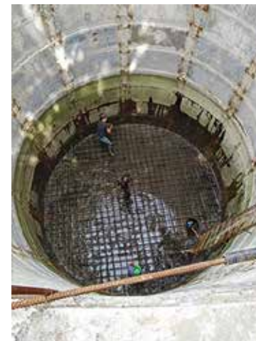
Figure 6.19. Reinforcing and concreting the bottom of the pit shaft
