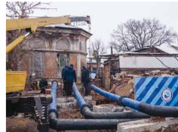
Figure 6.12. Arranging temporary wastewater disposal
