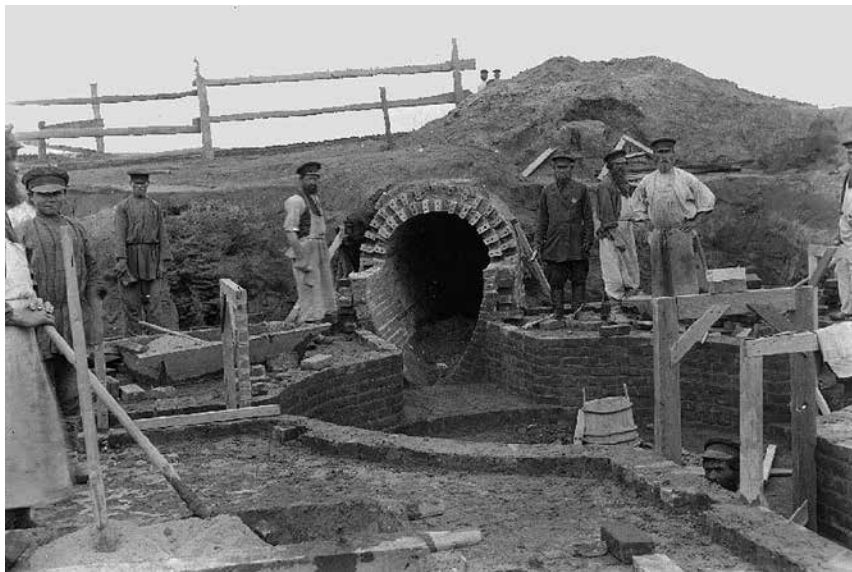
Figure 1.3. Construction of a brick sewer
