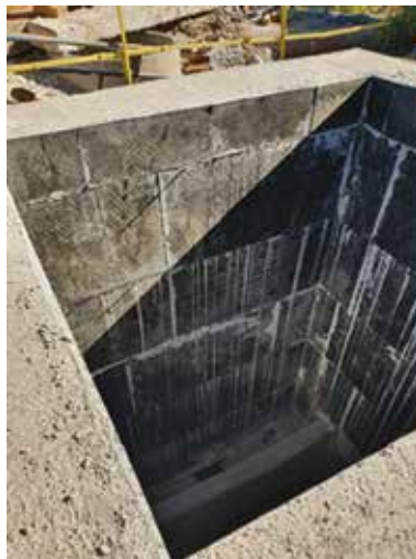
Figure 6.41. A pit shaft rehabilitated using PE sheets
