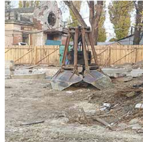
Figure 6.17. Excavating the invert part using the grab
