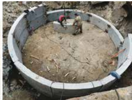
Figure 6.16. A shell ring of the future pit shaft
