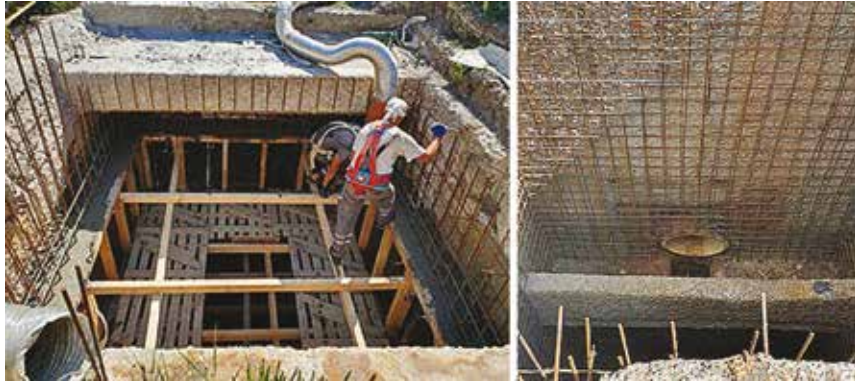
Figure 6.39. Restoring the geometry of the tunnel shaft
