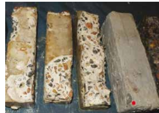
Figure 3.11. Uncoated and coated specimens after being exposed in the sewer for 140 days
