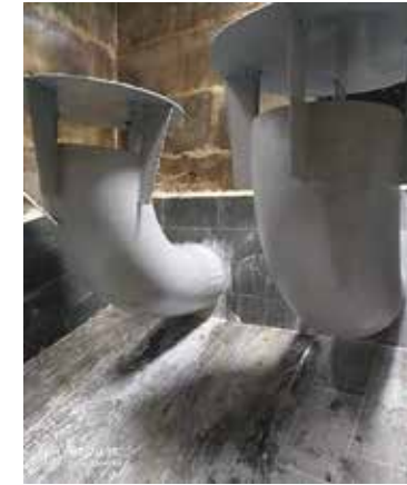
Figure 6.31. Stilling chamber K-1: general view after rehabilitation work
